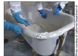
Workers use a methylene-based stripper to remove paint from a bathtub prior to refinishing.
