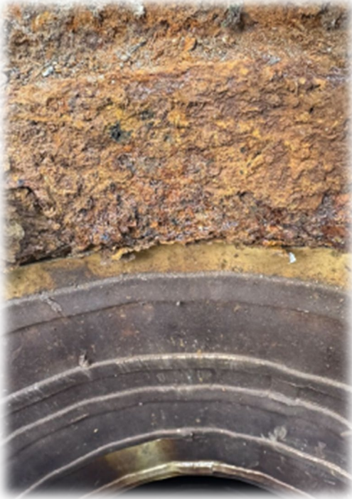
visual corrosion of barrels
