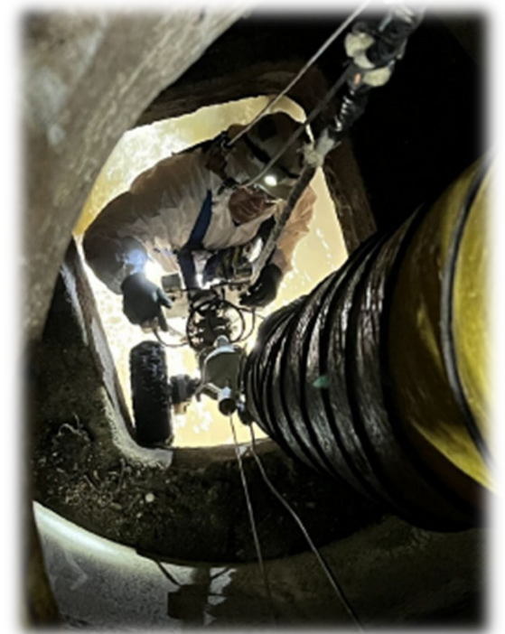
Manned entry required to configure laser ring on crawler in the pipe
