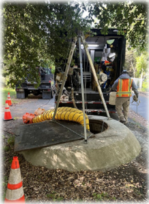
Tripod to raise/lower staff when setting up MSI equipment; supplied air to reduce condensation on camera
