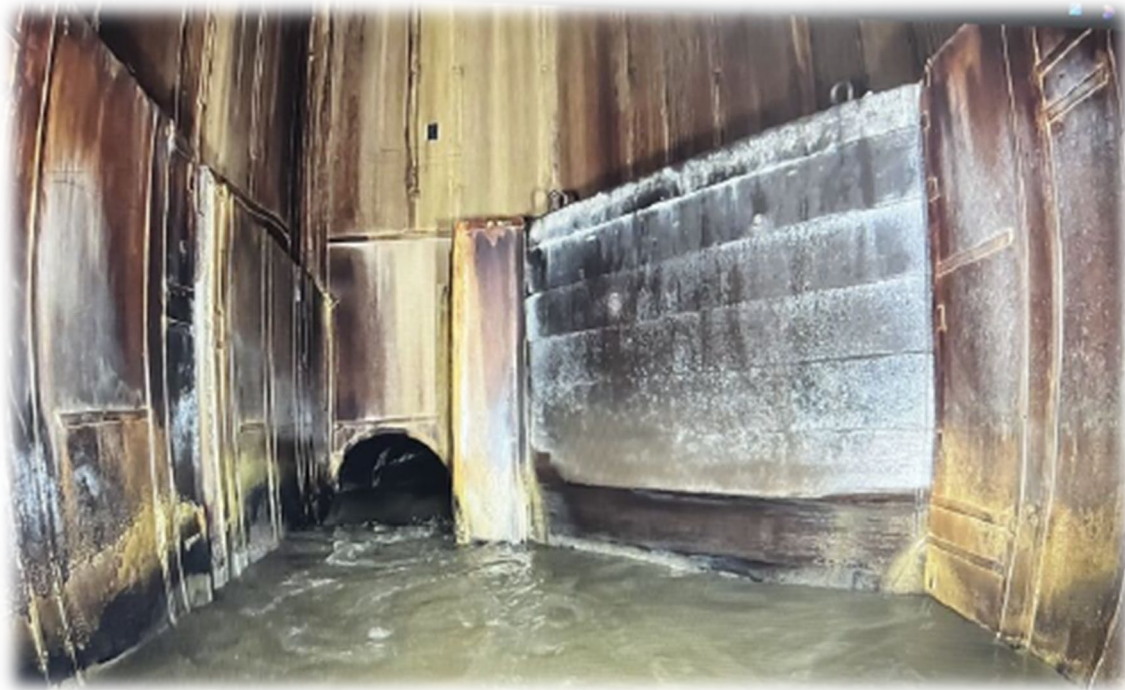
Confirm configuration of junction structures from CCTV
