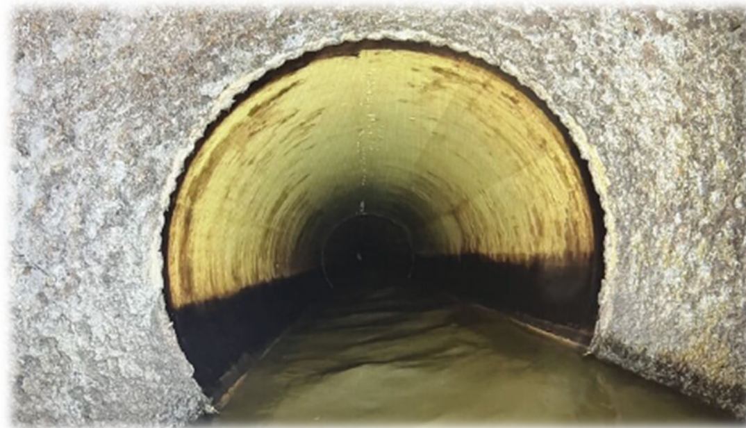
Unlined to lined, generally good (visual) condition
