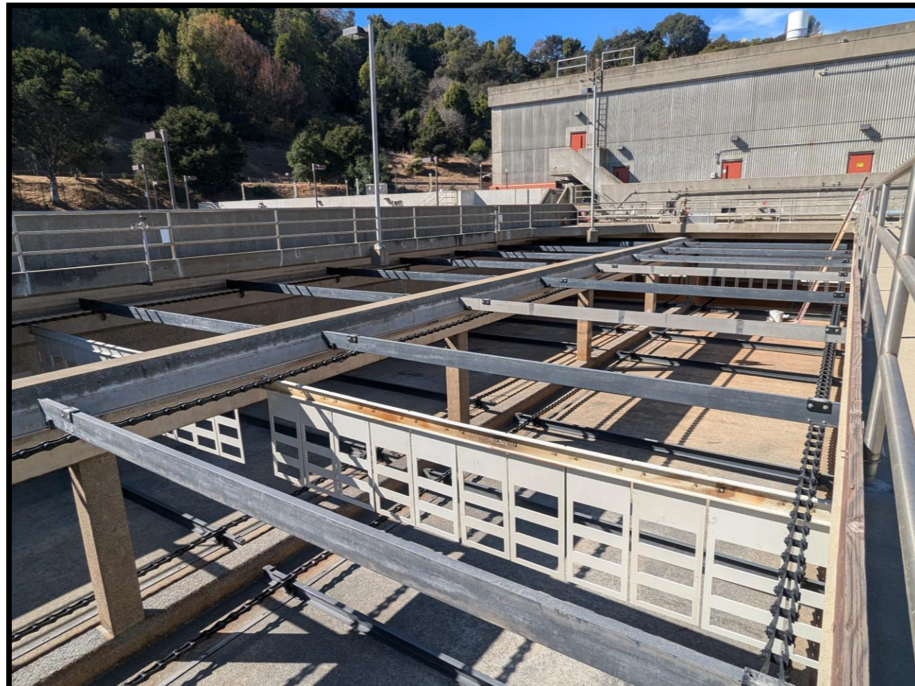
Flow Optimization Baffles Increase Organics Capture
