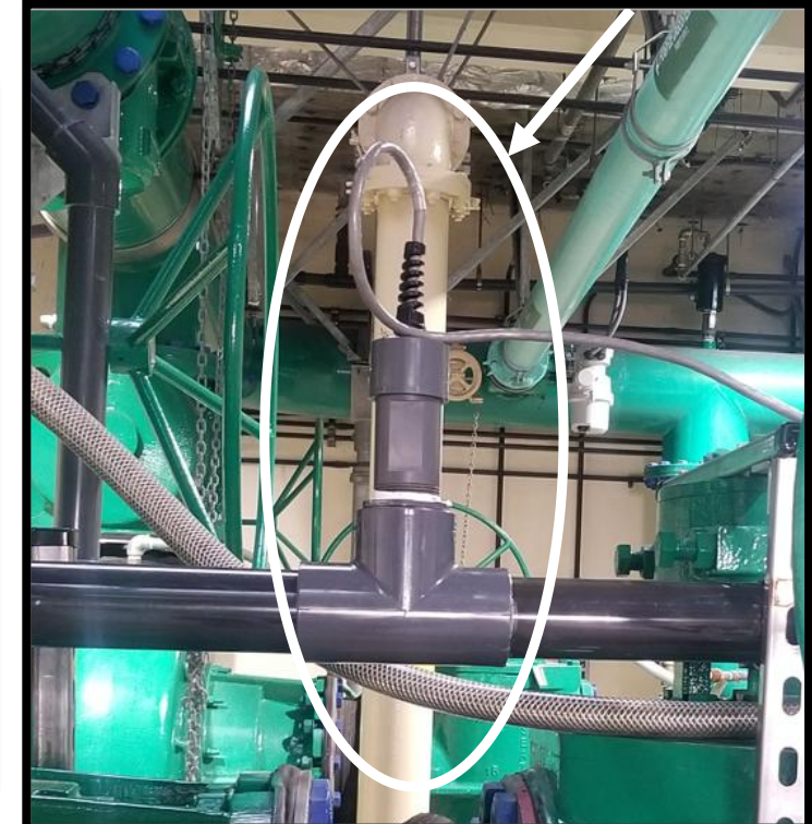
Sentry probes installed at digester recirculation pumps
