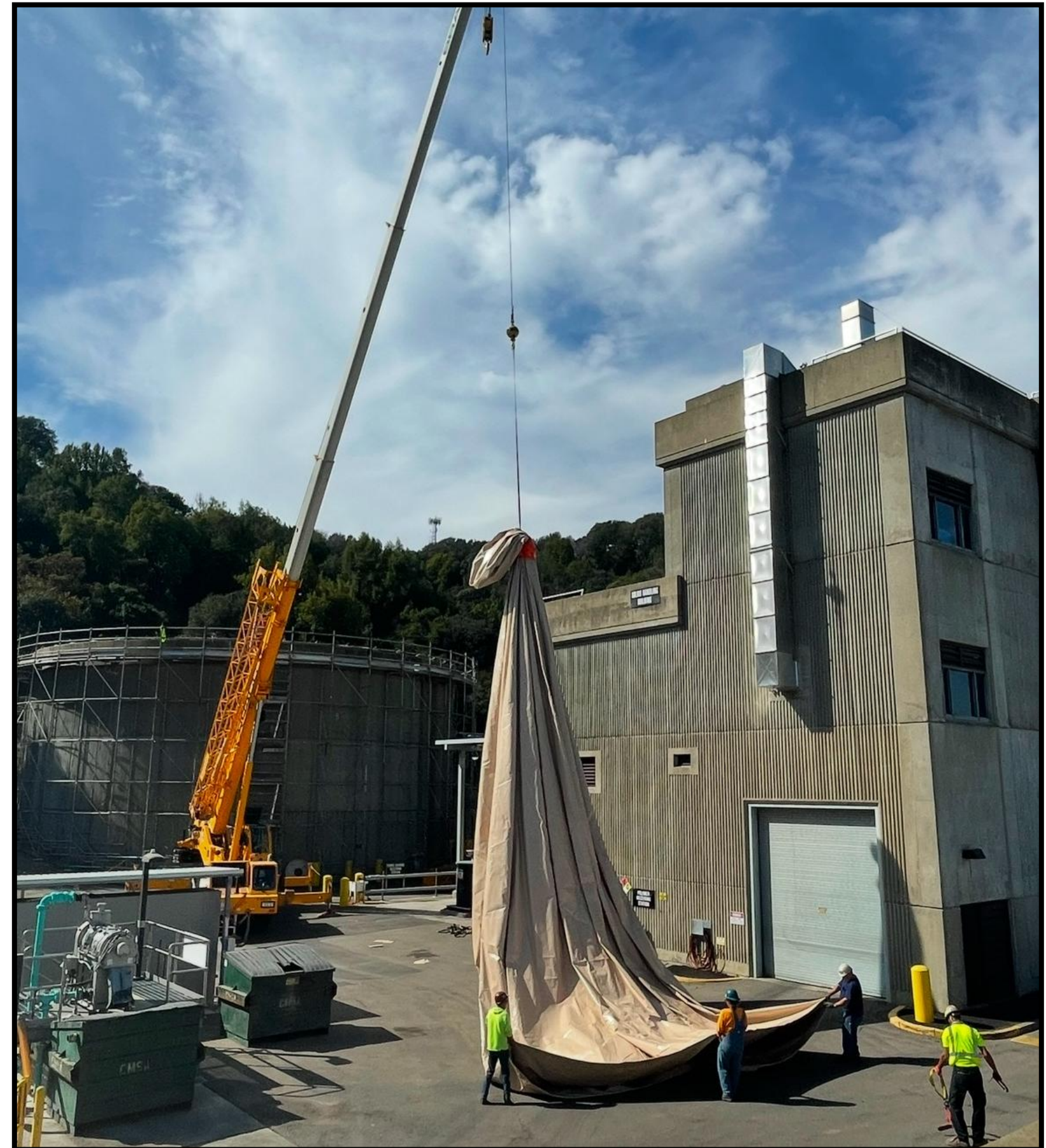
Digester Membrane Replacement
