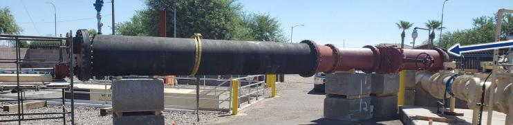
Inspection Prep: Install temporary launch piping
