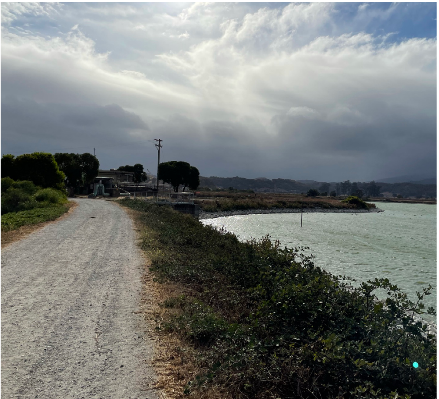
Levee and storage pond.
