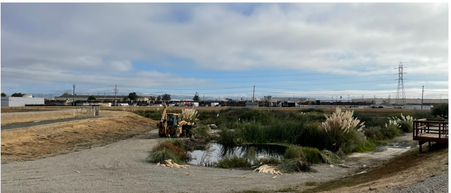
Vegetation removal at the dual purpose basin in 2023.
