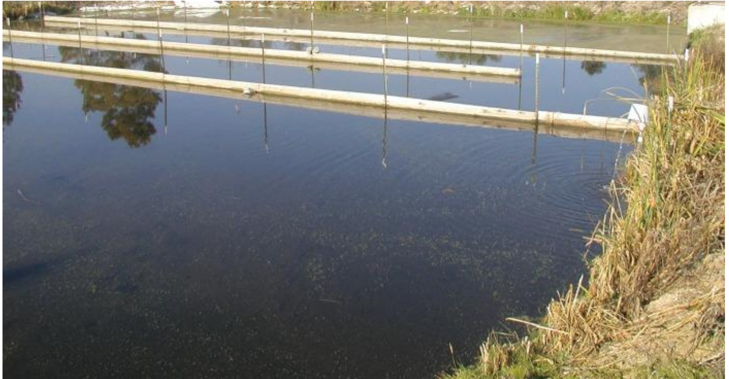
Figure 4. Picture of Discovery Bay Open-Water Wetland Cell Located in Discovery Bay, CA) (Jasper et al., 2013)
