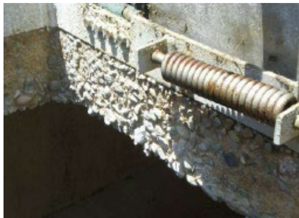
Significant issues with concrete roof of Existing Aeration Basins 1-4 (1978)
