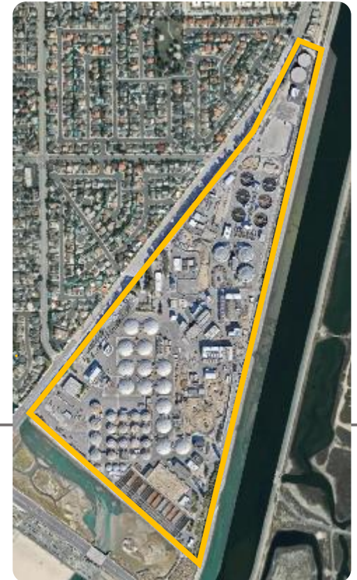
Treatment Plant No. 2 Huntington Beach
