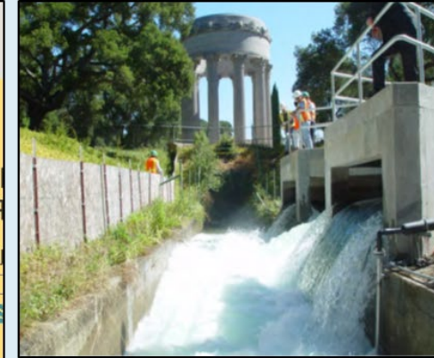
Above: Flows from the Pulgas Dechlorination Facility enter the Pulgas Discharge Channel for release to Upper CSR.
