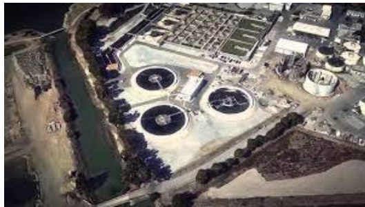
Oro Loma SD 80% TIN removal from influent
