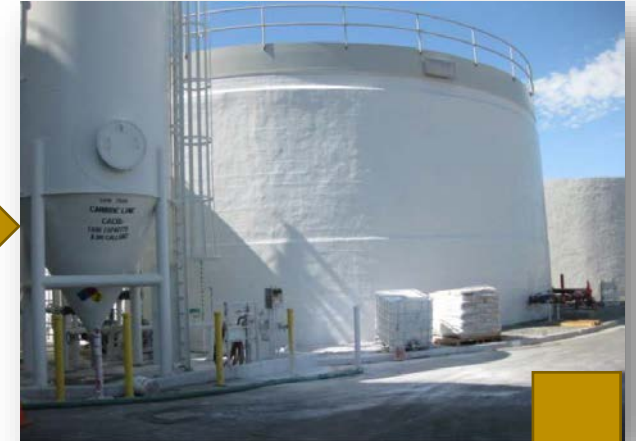
Sludge Blending Tank
