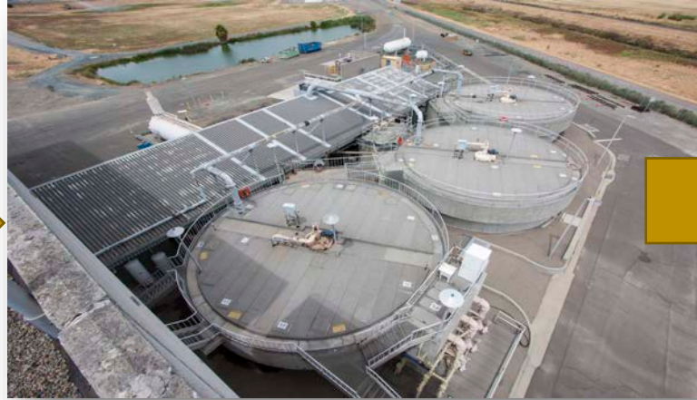
Dissolved Air Flotation Thickener
