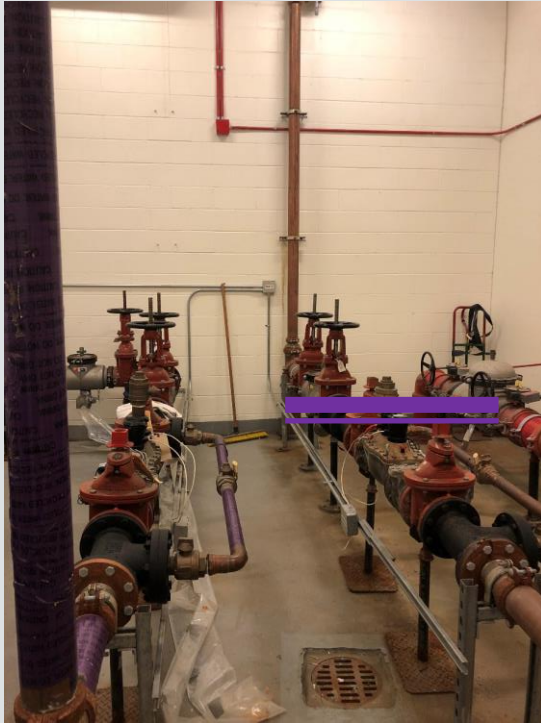
RW and Potable Water Backflows
