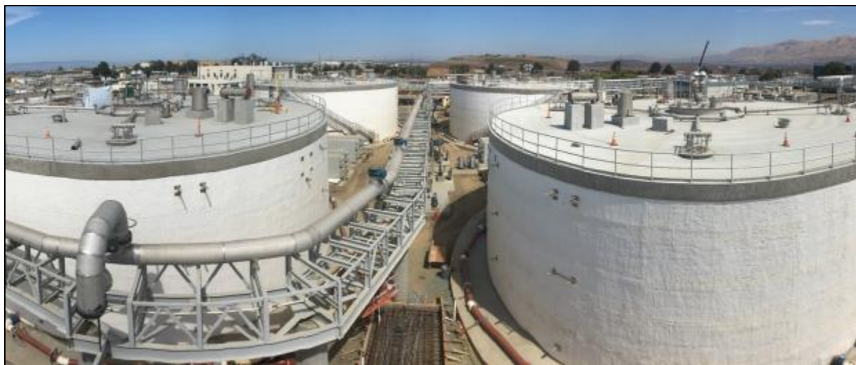
Photo: Upgraded Digesters for Temperature Phased Anaerobic Digestion at San José-Santa Clara Treatment Plant. Source: City of San José .
