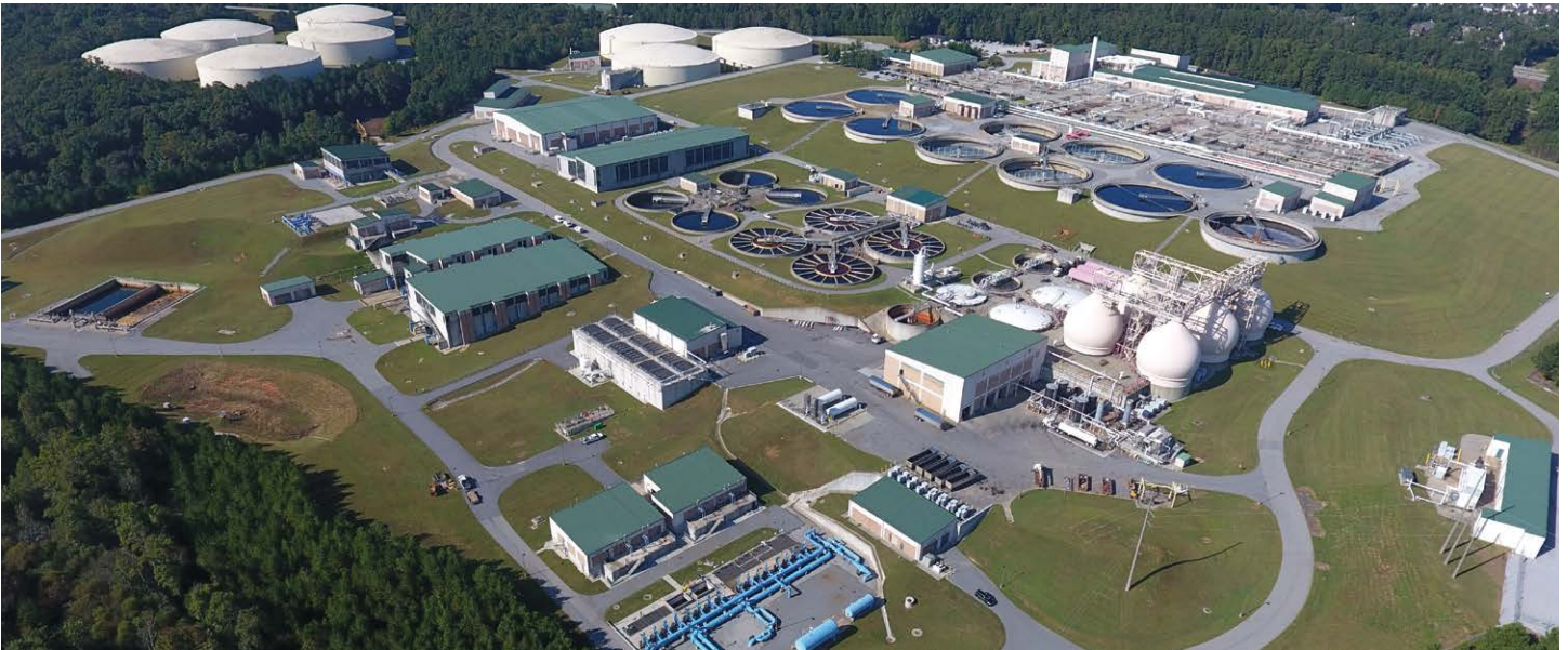
The F. Wayne Hill Water Resources Center in Gwinnett County, Georgia, treats up to 60 MGD of wastewater effluent for surface water recharge to Lake Lanier, while also recovering phosphorus and methane gas.
