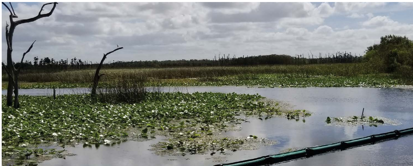
Constructed wetlands in Orlando, Florida, provide advanced treatment for reclaimed water.
