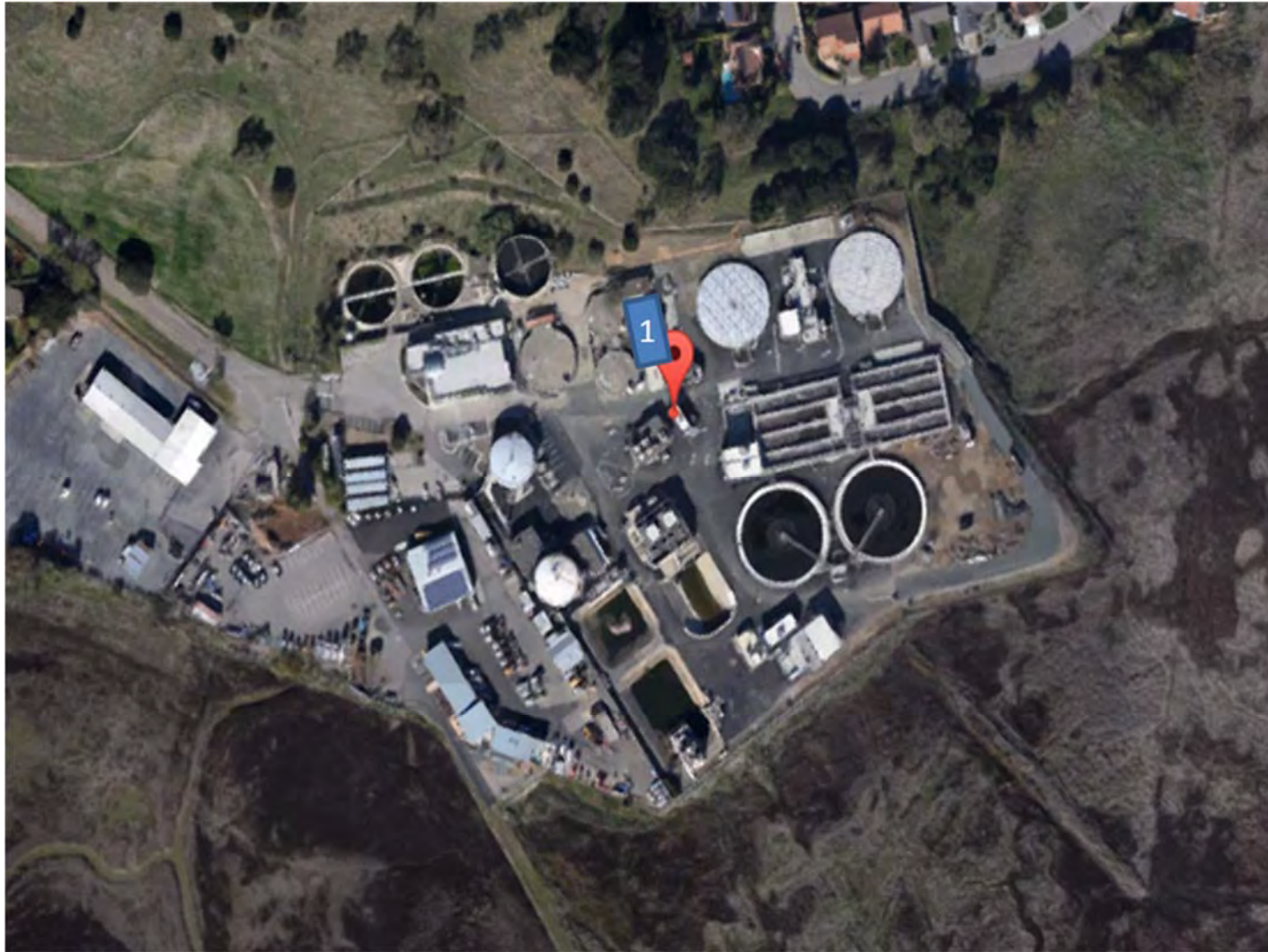
Figure 6-3. Level 2 Upgrade Aerial Layouts for Dry Season and Year Round (1) chemical addition facilities (alum and methanol).
