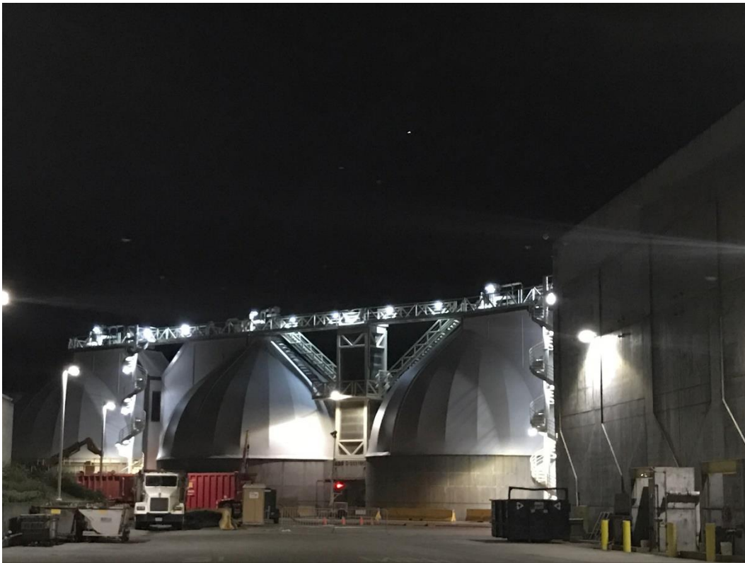
Photo: Anaerobic Digesters at San Francisco's Oceanside Wastewater Plant
