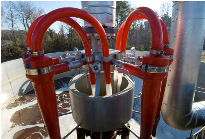
Figure 17. Image of DEMON ® Hydrocyclone at HRSD York River Plant.
