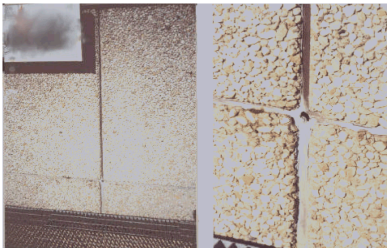
Figure B-1. Caulking compound in an expansion joint of a concrete structure.
