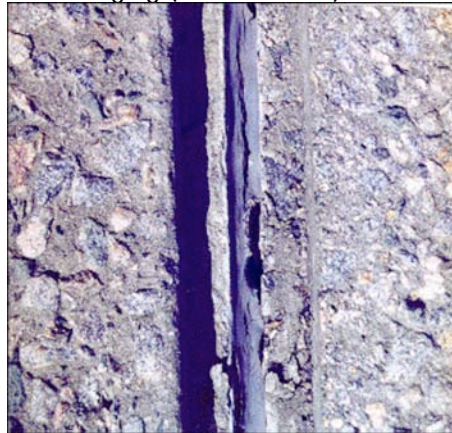
Figure B-1. Caulking compound in an expansion joint of a concrete structure.
