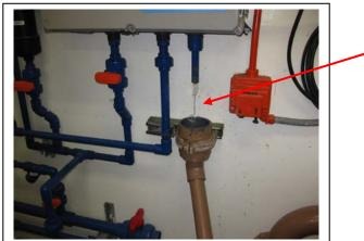
This is an example of a continuous flow sampling port to collect wastewater effluent for Dioxins/furans testing. Assemble the following containers:
