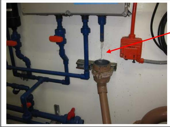
This is an example of a continuous flow sampling port to collect wastewater effluent for Dioxins/furans testing. Assemble the following containers:
