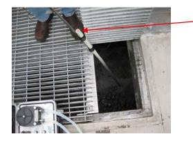
Suspend the flexible tubing through a PVC conduit to assure the depth is 6-12 inches below the water surface. Loose tubing will skip on the surface of the flow with no weight to hold it under
