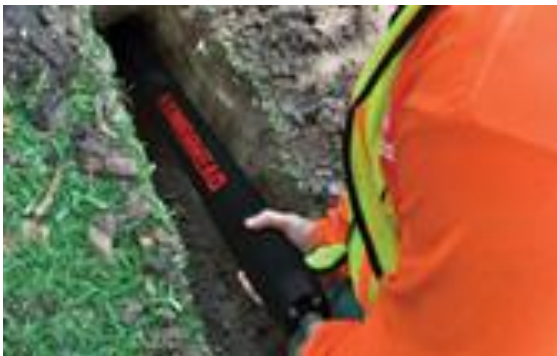
Piercing Equipment Photo courtesy of Ditch Witch
