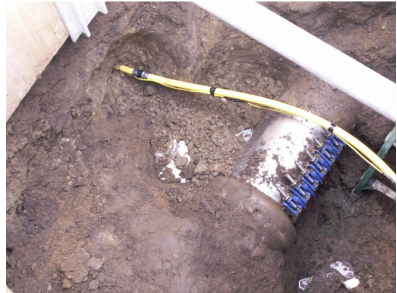
Relocated gas line
