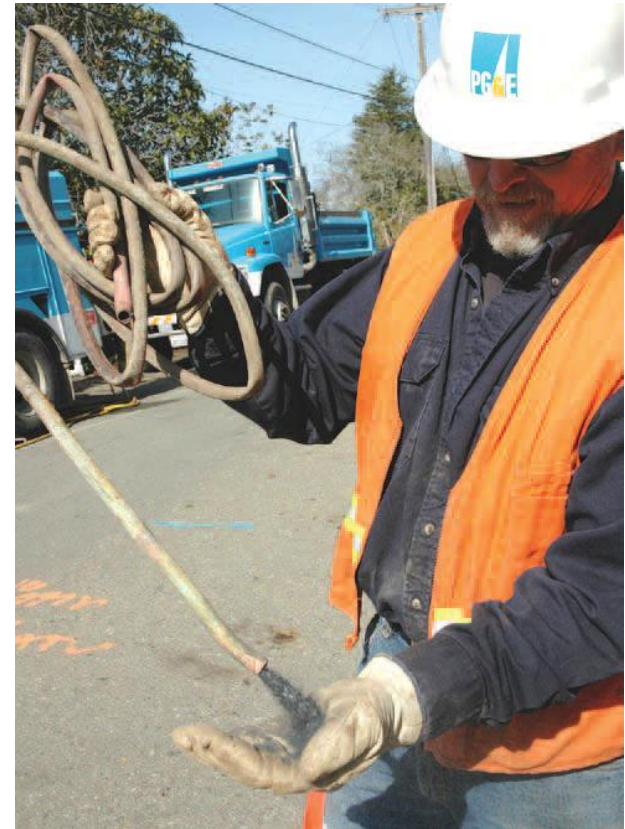
Tom Blum shows the flakey evidence of corrosion in the copper pipe.
