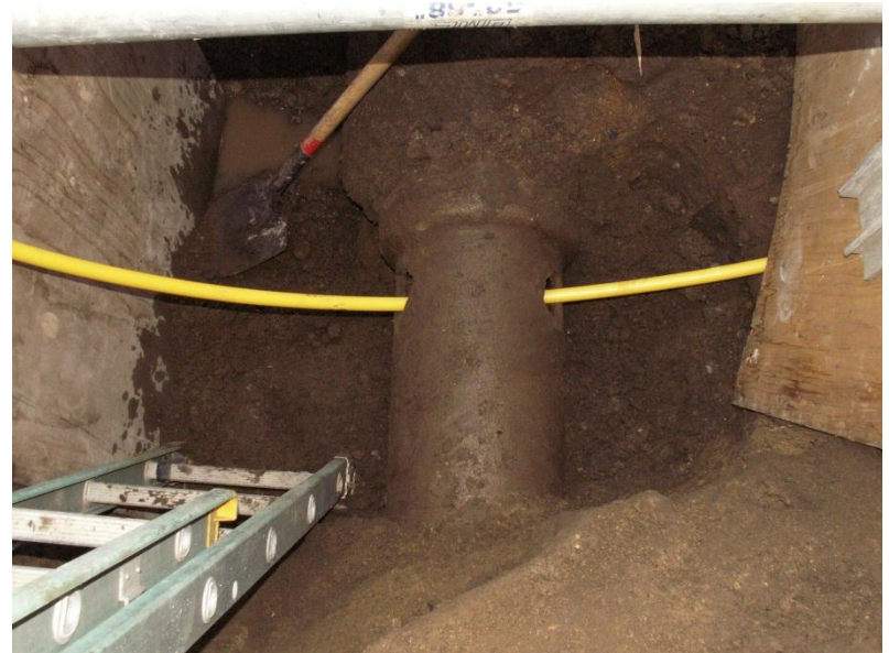
Excavated cross bore
