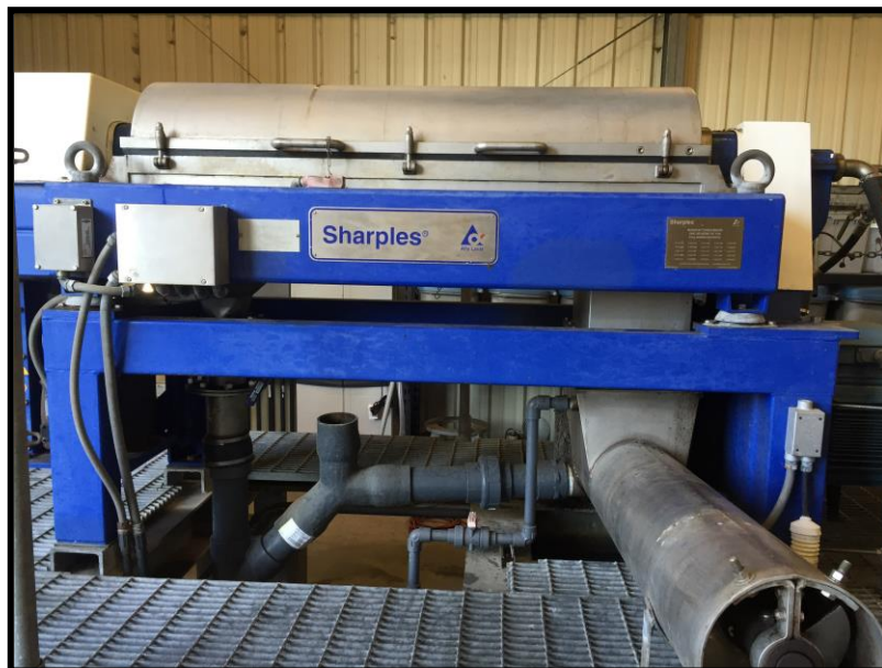
Centrifuge Unit at Rancho Santa FE WRF - San Diego County
